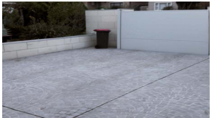
Synthetic stone covering (3 cm thick)
