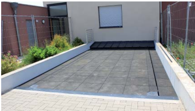
Rubber covering in stone structure (3 cm thick)
