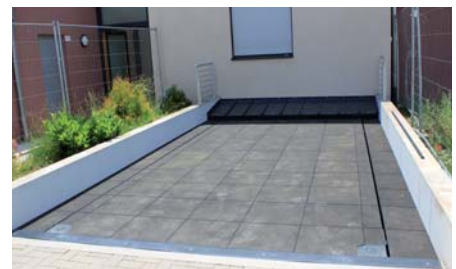
Rubber covering in stone structure (3 cm thick)
